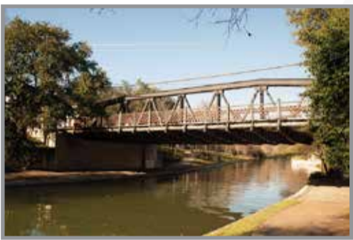
ARSENAL ST BRIDGE
