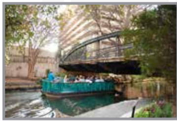
NUOVA ST BRIDGE
