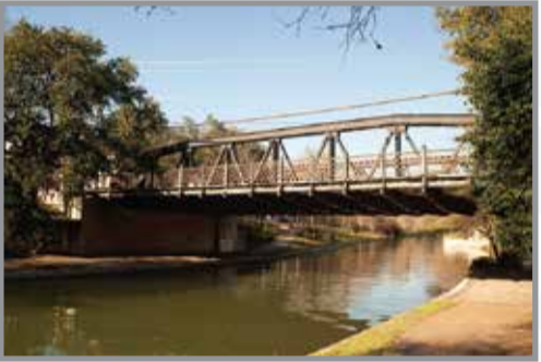
ARSENAL ST BRIDGE
