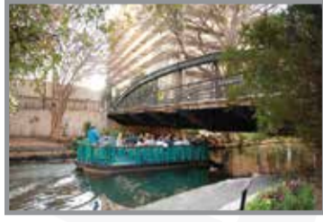
NUOVA ST BRIDGE
